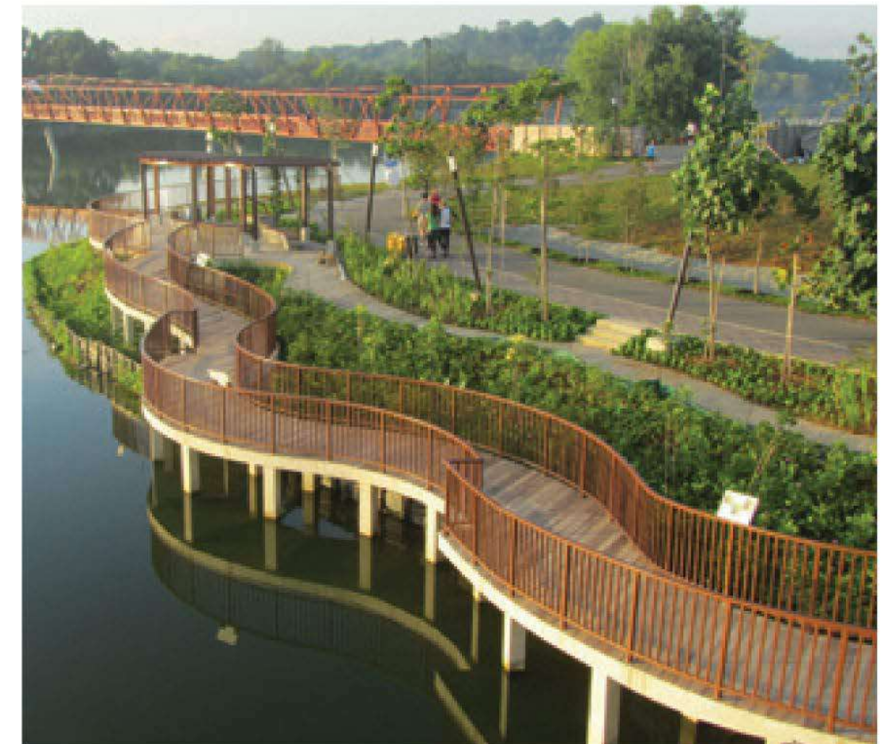
PUNGGOL WATERWAY, SINGAPORE
